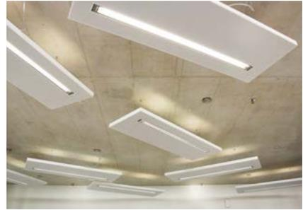
The building does not feature a traditional suspended ceiling, but acoustic panels with lighting fixtures in them. The use of such panels allows for ‘concrete core activation’, which means that the thermal mass of the building’s concrete structure is used to regulate the indoor climate. (photo: Royal HaskoningDHV)
