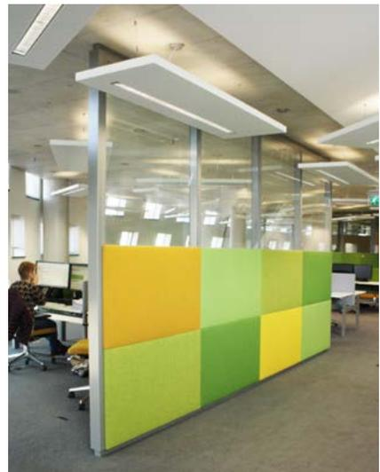
Partitions divide the open plan office into smaller parts. The lower part of the partition consists of sound absorbing panels. The upper part is glazed, which helps to maintain a sense of openness and allows daylight to penetrate the inner parts of the building. (photo: Royal HaskoningDHV)
